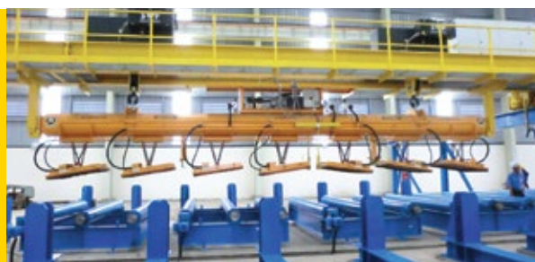
25-ton x 16m gantry crane, PV Pipe, Go Cong Town, Tien Giang Province
